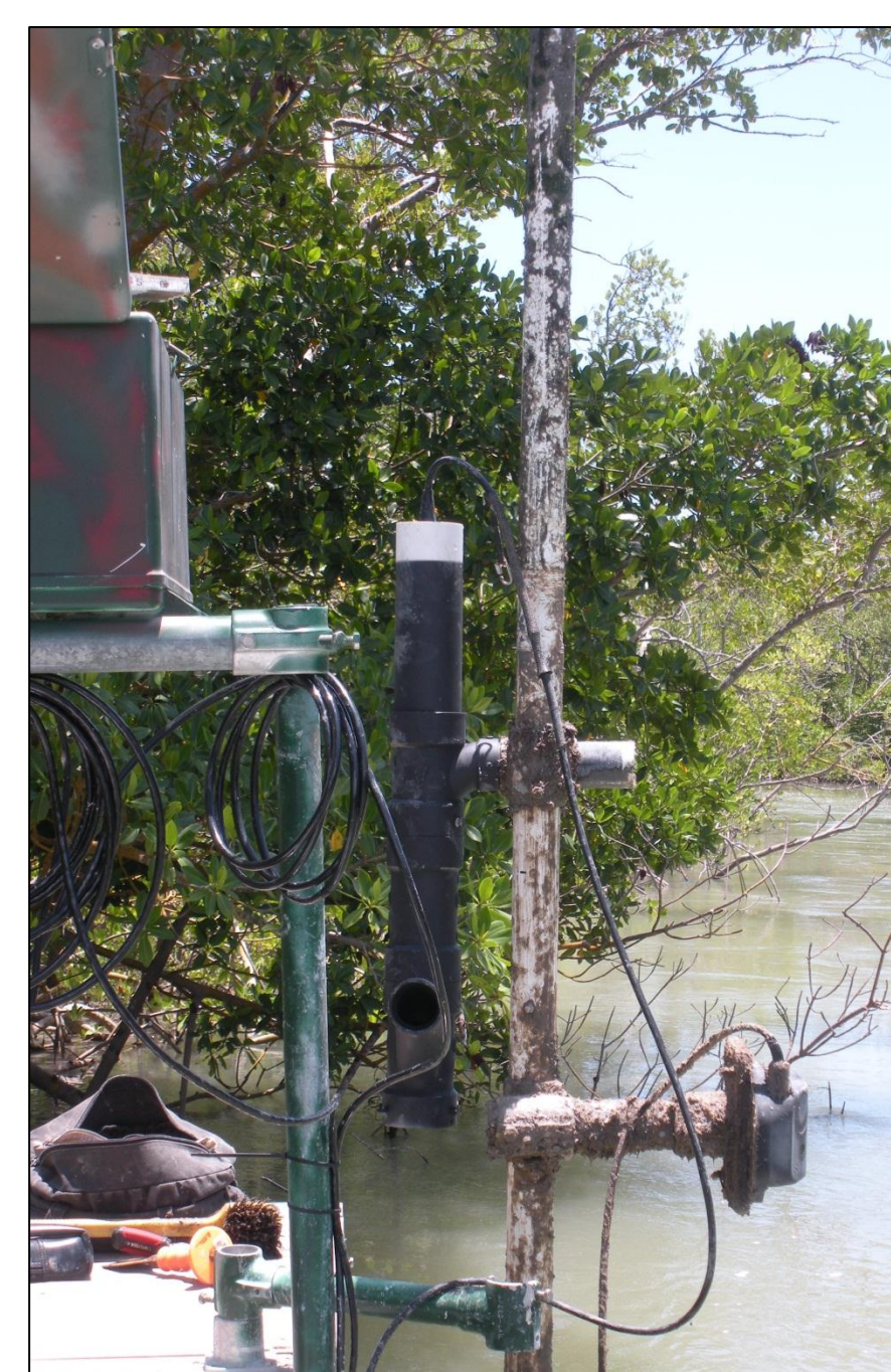
Photograph of the YSI and Sontek SL equipment mounts out of the water during a routine servicing.
