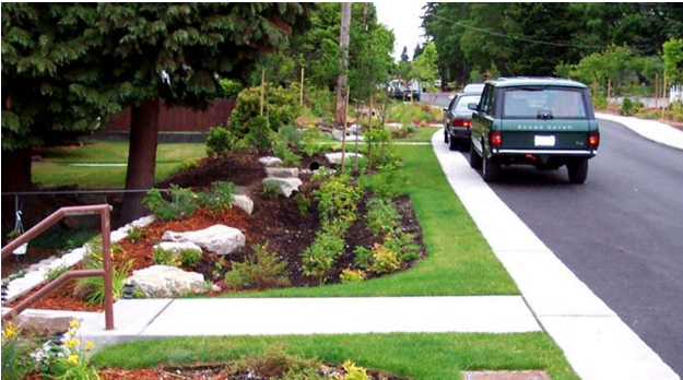
Bioswales are landscaping features that slow and collect polluted stormwater runoff where it will infiltrate soils and be treated by natural elements.
