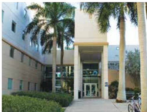
INDIAN RIVER TOWERS
