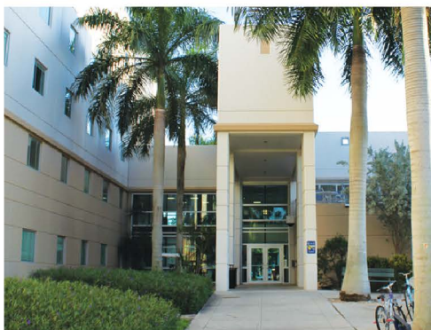
INDIAN RIVER TOWERS
