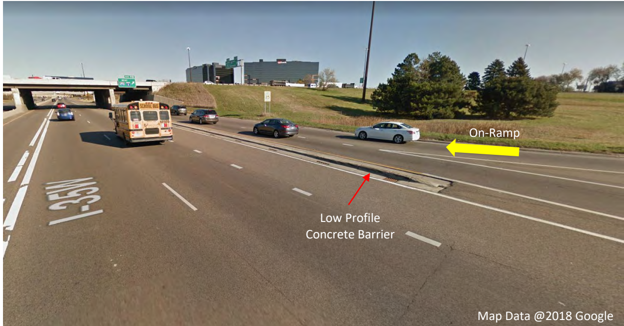
(b) I-35W NB at I-494 Interchange in Bloomington, MN Figure 30: Example of Barrier to Separate On/Off-Ramp Traffic from Mainline
