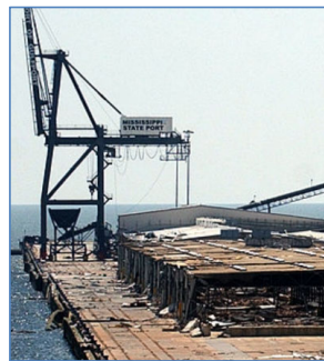
Port Structures and Facilities
