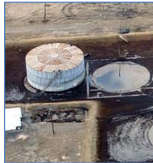
Above Ground Storage Tanks
