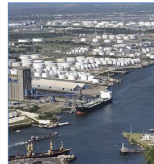
Industrial Complexes and Communities
