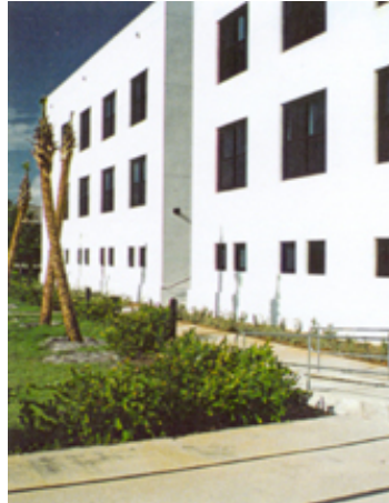
Incorrect: Little Shading and Arcading
