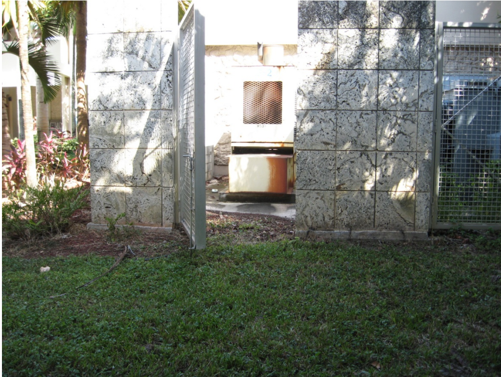
400-gallon, double-walled diesel belly tank.
