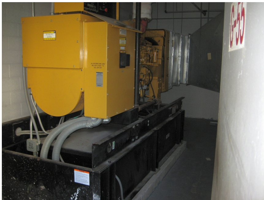
400-gallon, double-walled diesel belly tank.
