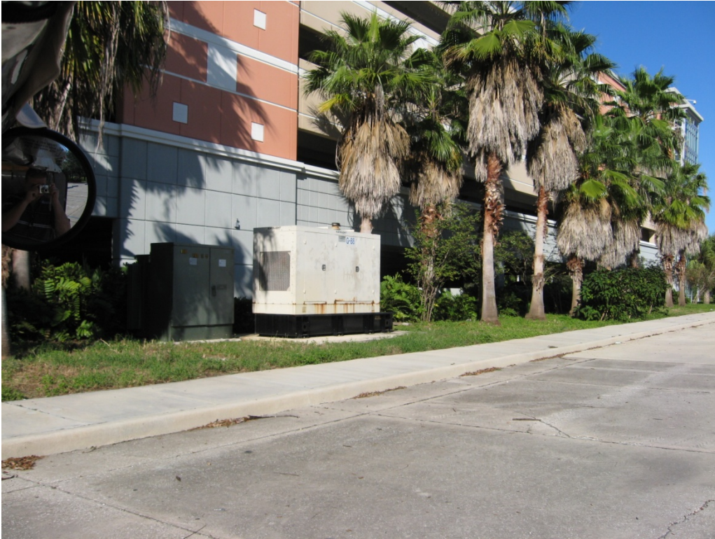
250-gallon, double-walled diesel belly tank.
