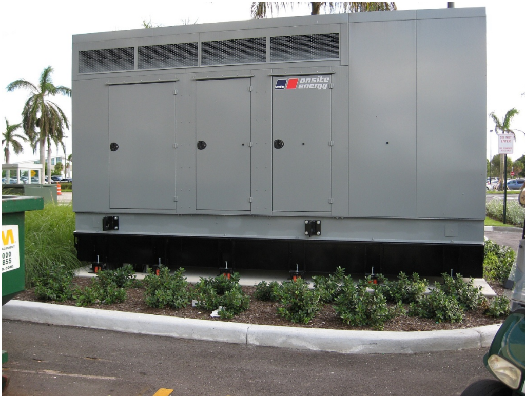
650-gallon, double-walled diesel belly tank with electronic interstitial monitoring and no drain plug.
