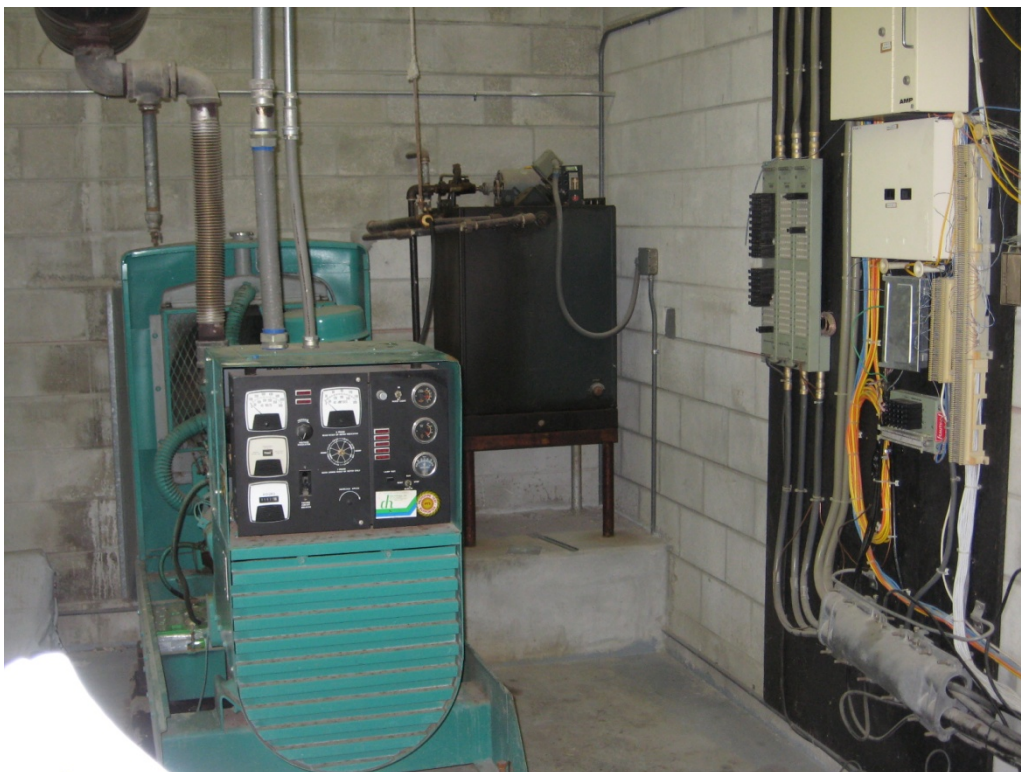
250-gallon, double-walled diesel belly tank.
