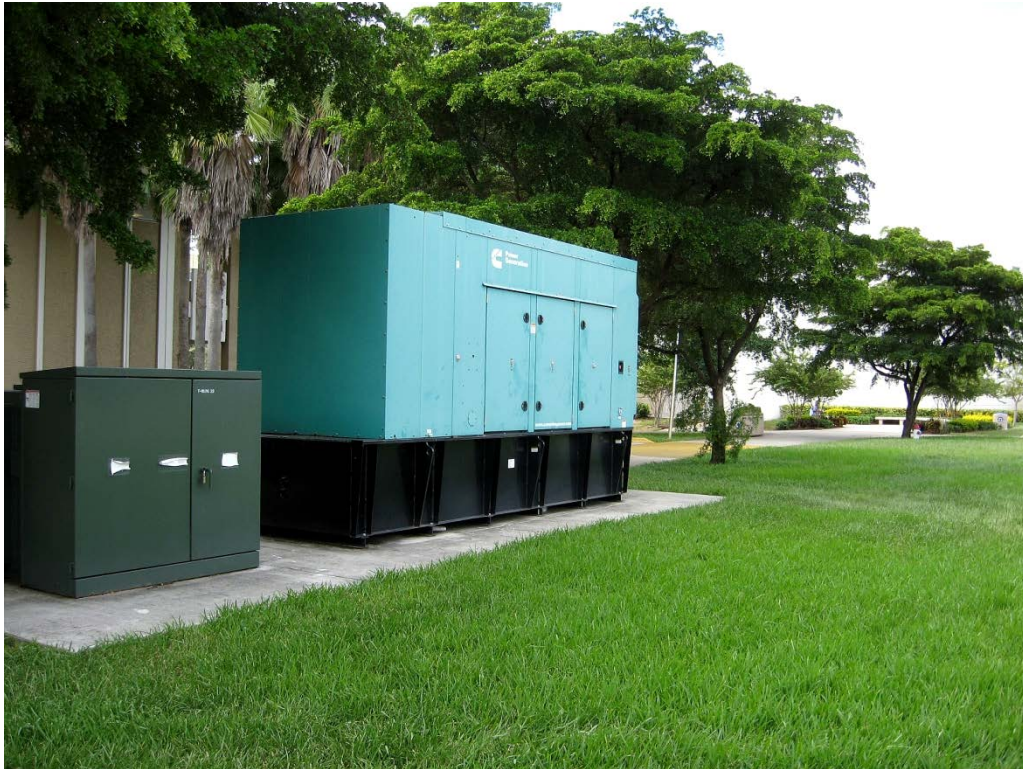
1,700-gallon, double-walled diesel belly tank with interstitial drain.
