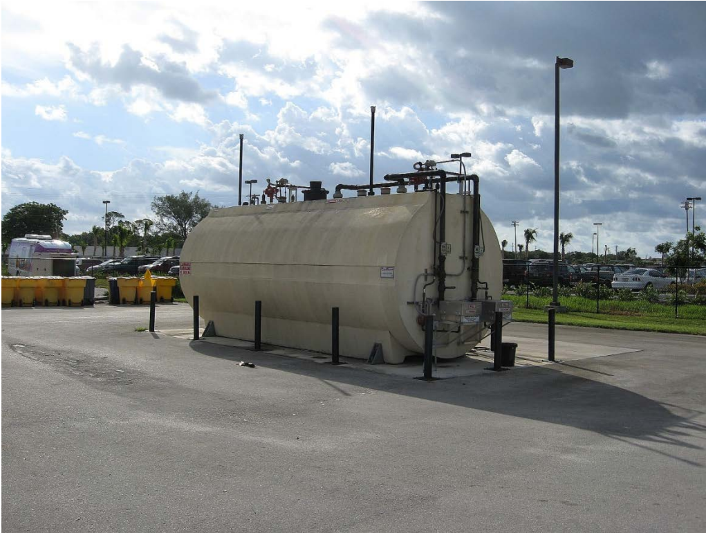
5,000-gallon gasoline/3,000-gallon diesel, double-walled AST with (2) "Greenleaf" electronic level & interstitial monitoring gages, Model EFG-8000
