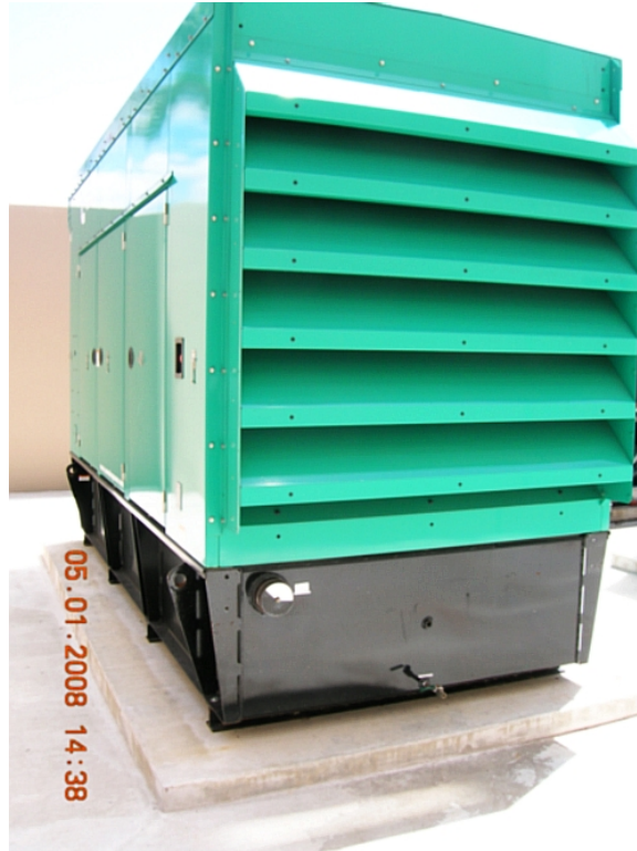
850-gallon, double-walled diesel belly tank with interstitial drain.
