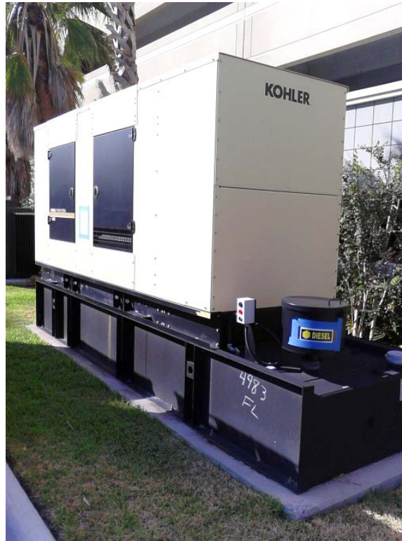
555-gallon, double-walled diesel belly tank with electronic interstitial monitoring and no drain plug.
