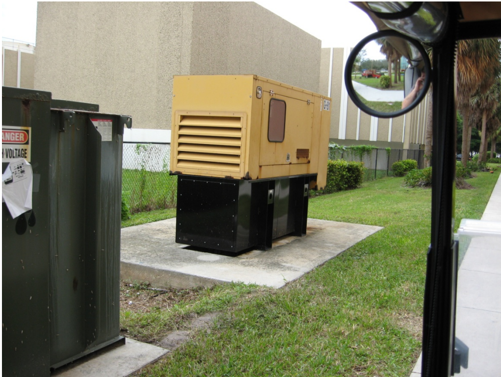
250-gallon, double-walled diesel belly tank.
