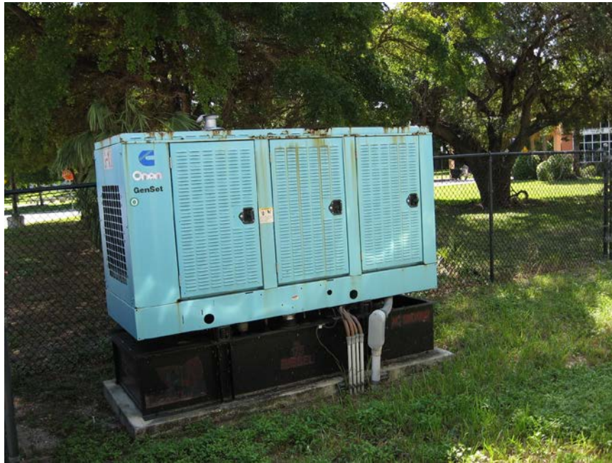
175-gallon, double-walled diesel belly tank.
