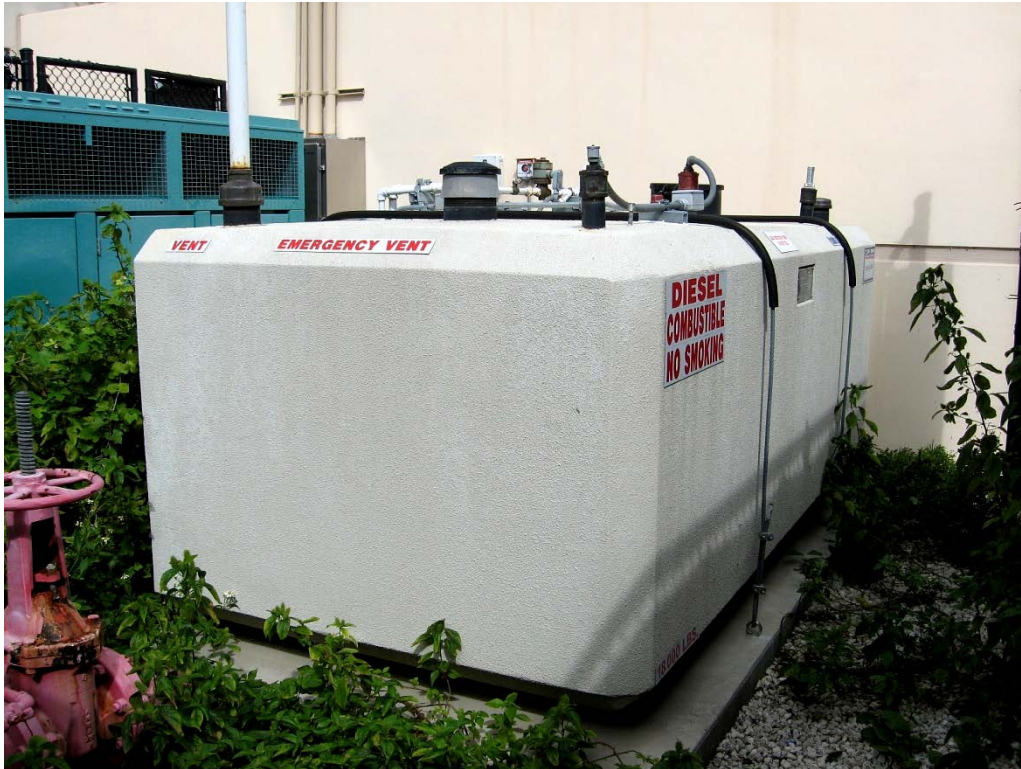
1,000-gallon, double-walled, vaulted diesel tank with electronic interstitial monitor.
