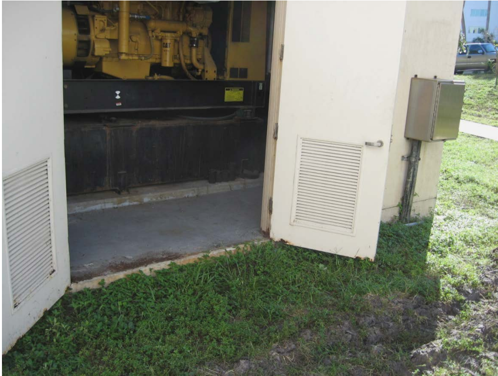
400-gallon, double-walled diesel belly tank.
