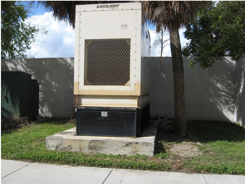
475-gallon, double-walled diesel belly tank.
