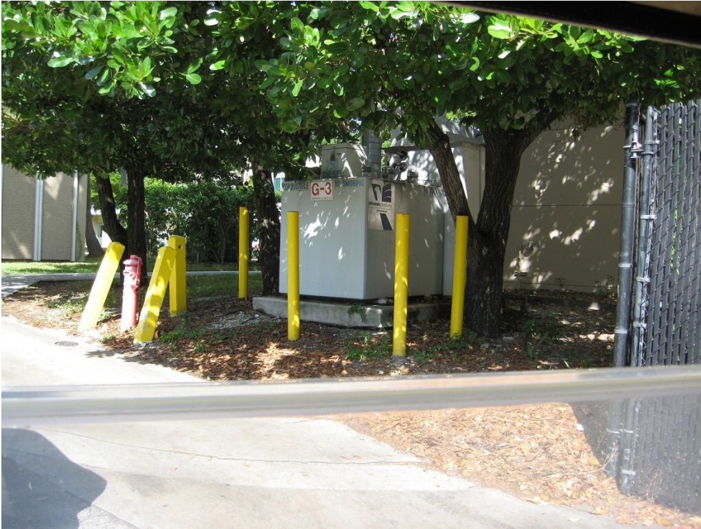
250-gallon, double-walled diesel belly tank.
