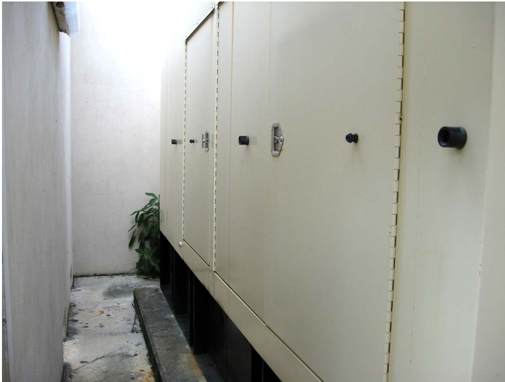
600-gallon, double-walled diesel belly tank with electronic interstitial monitoring.
