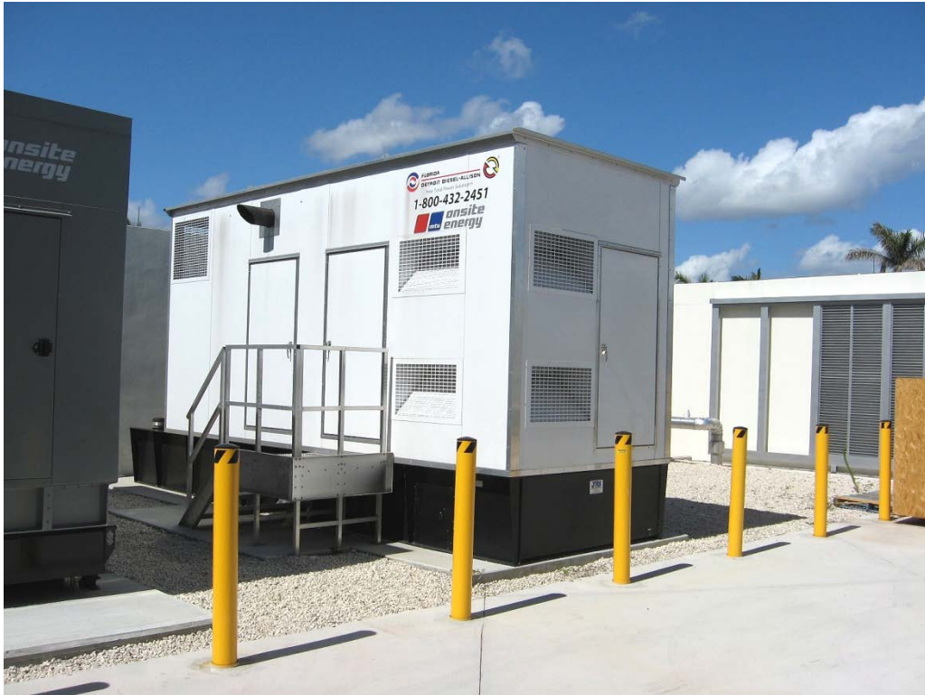
2,200-gallon, double-walled diesel belly tank with electronic interstitial monitoring and drain plug.
