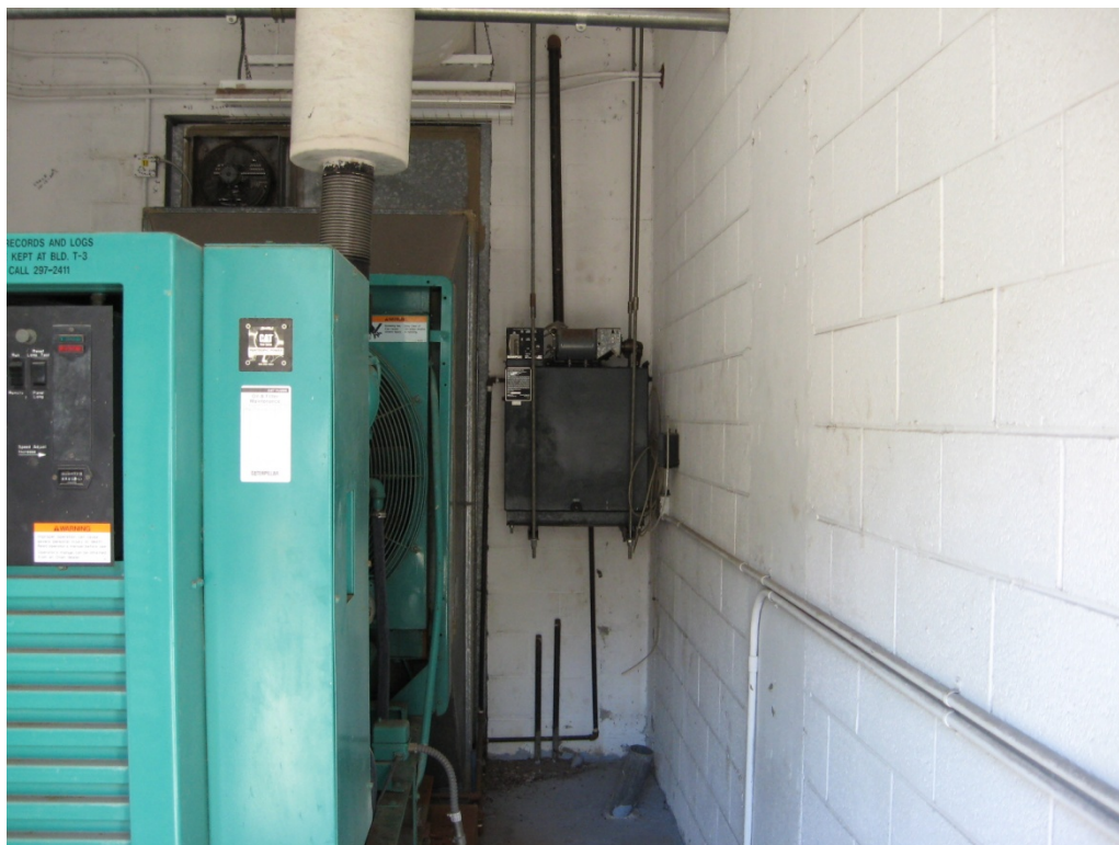
250-gallon, double-walled diesel belly tank.
