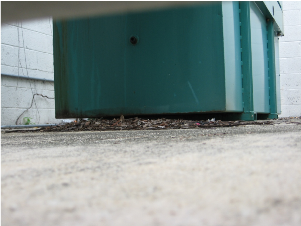
366-gallon, double-walled diesel belly tank.
