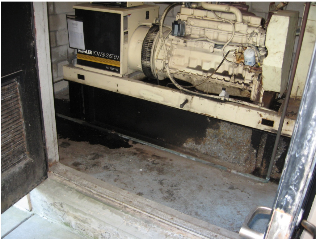
250-gallon, single-walled diesel belly tank.
