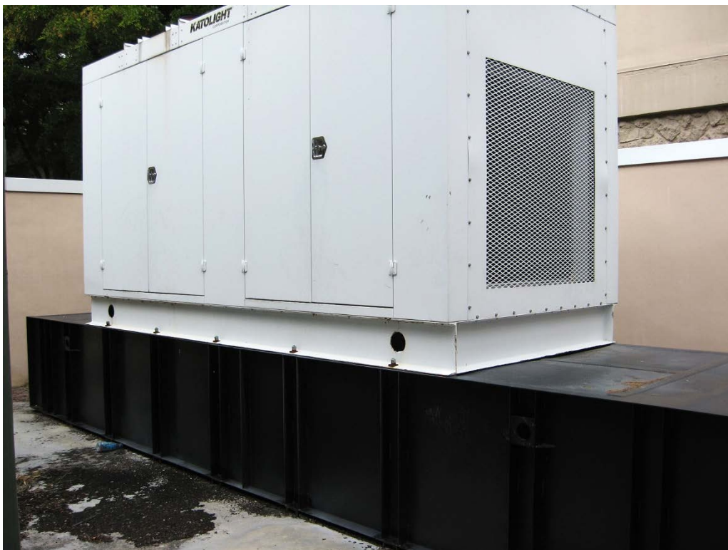
2,000-gallon, double-walled diesel belly tank with Krueger interstitial leak gage.
