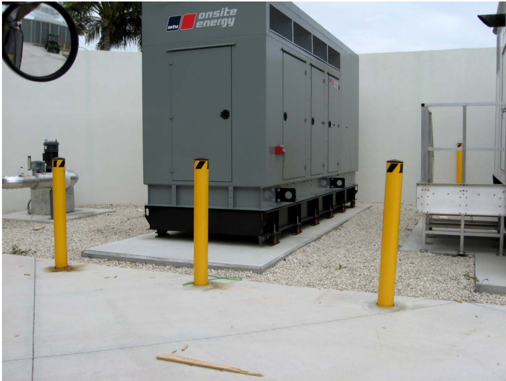
500-gallon, double-walled diesel belly tank.
