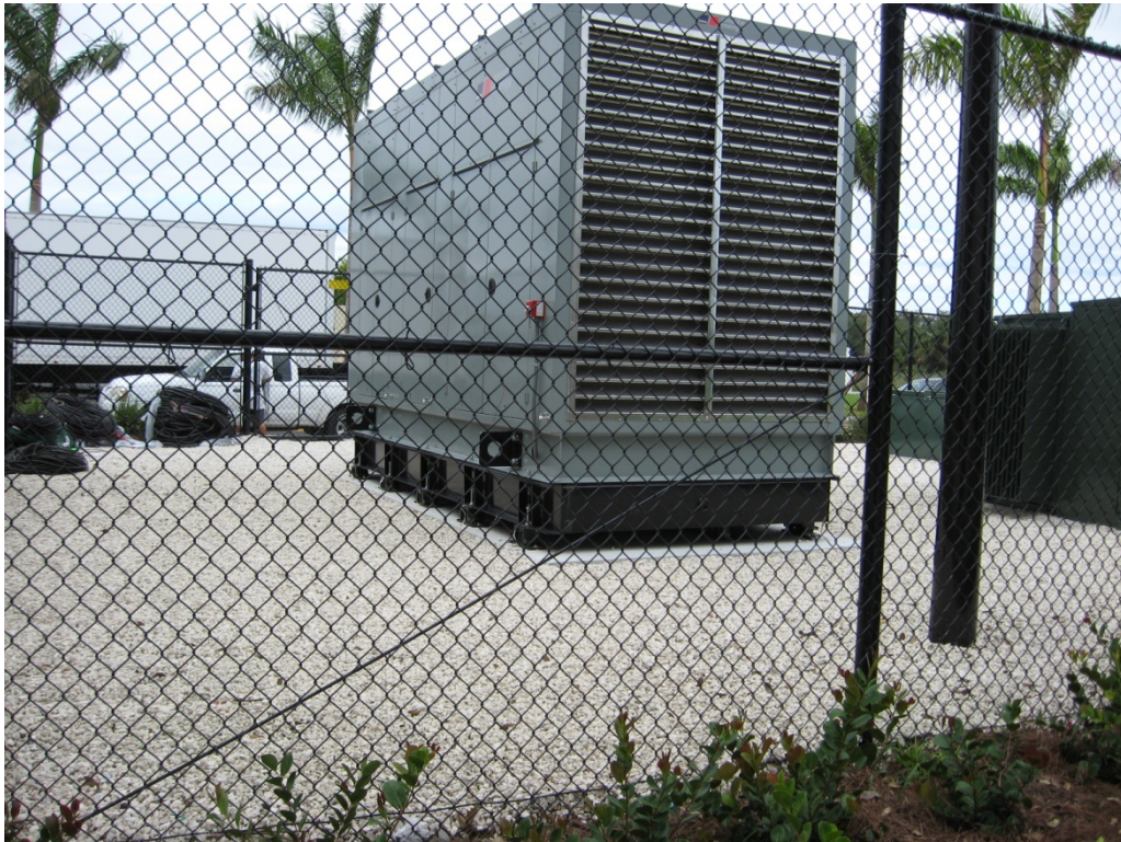
450-gallon, double-walled diesel belly tank.
