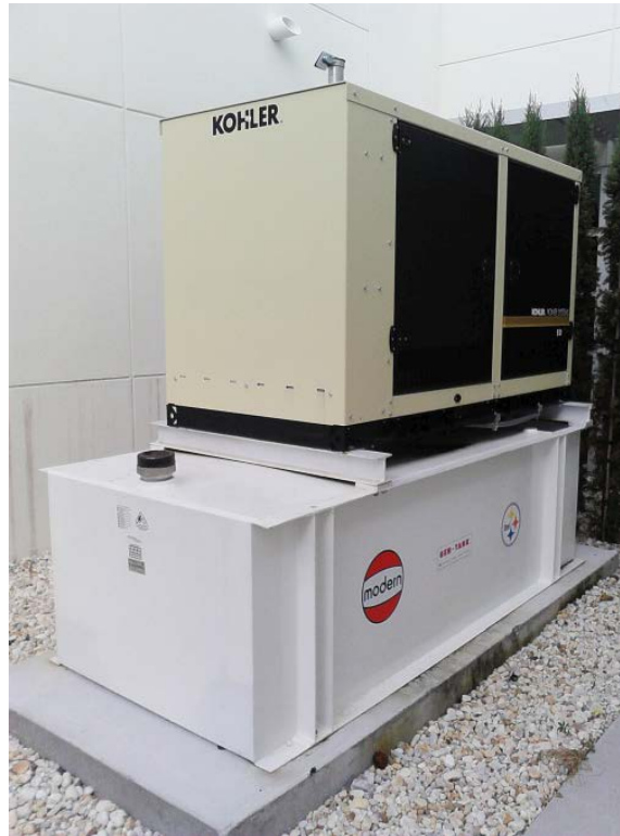
200-gallon, double-walled diesel belly tank.
