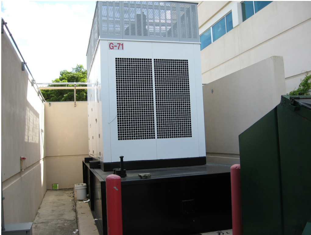
3,000-gallon, double-walled diesel belly tank with interstitial drain.
