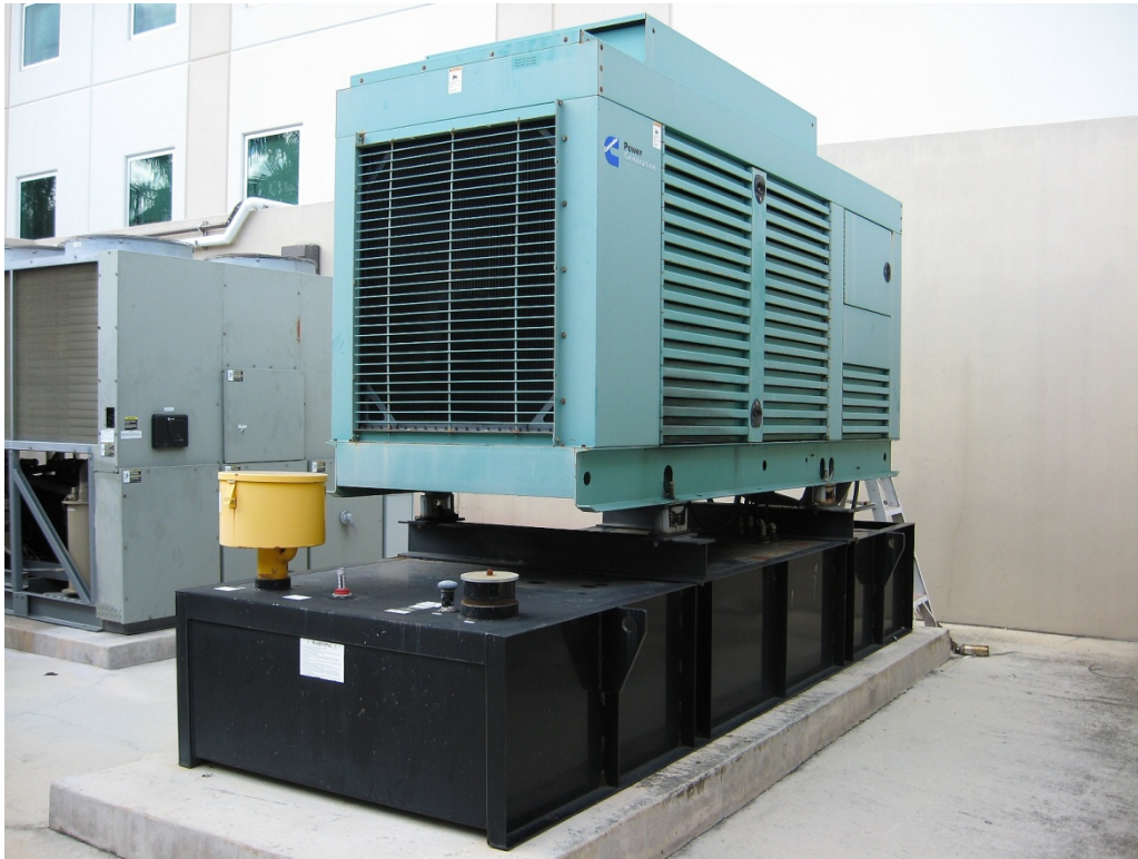
700-gallon, double-walled diesel belly tank with interstitial drain.
