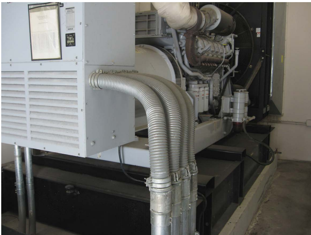
650-gallon, double-walled diesel belly tank with interstitial drain.
