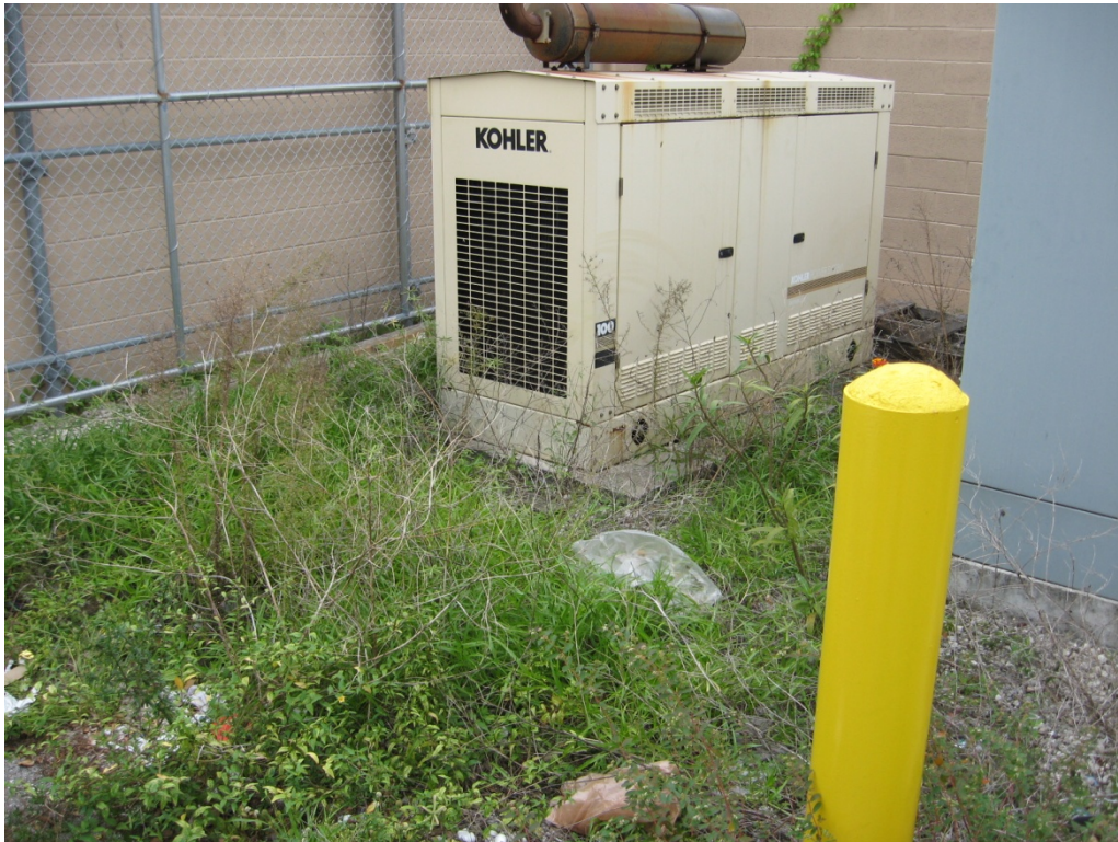
130-gallon, double-walled diesel belly tank.
