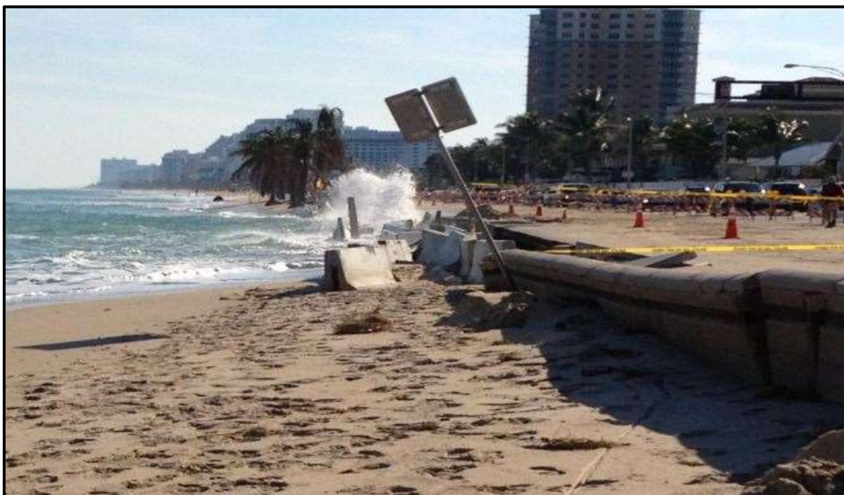
Figure 1. High energy waves damage beach, seawall, and road in Fort Lauderdale (Nov 2012, Keren Bolter)
