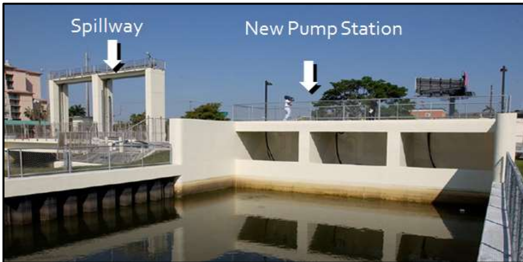
Figure 6. Adapted flood control structure in Miami-Dade County.
