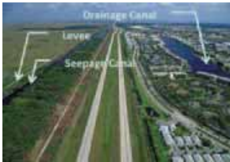
Figure 3. Water Control System
