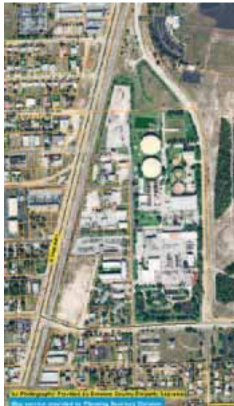
Figure 11. Water treatment plant in the City of Pompano Beach
