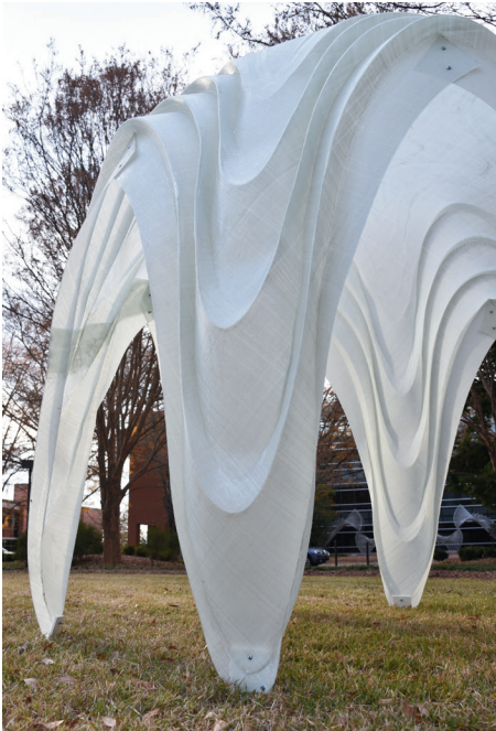
Photograph of the folded fiberglass vault.
