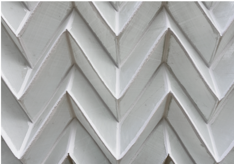
Photograph of the folded fiberglass tessellation on the side of the cube.
