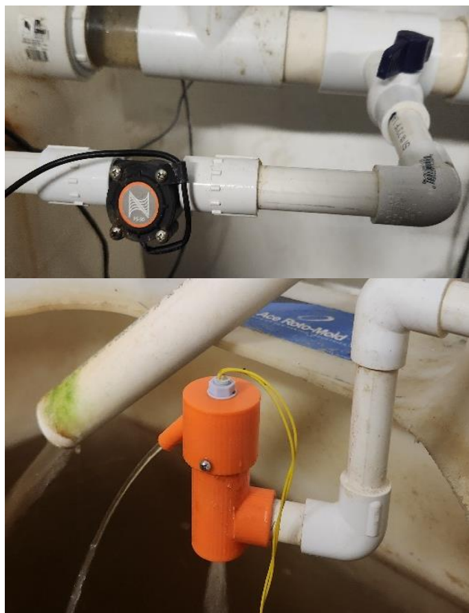
Figure 22. Example flow sensor installation of paddle wheel type flow sensor (top) and HBOI 3D printed float switch flow sensor (bottom).
