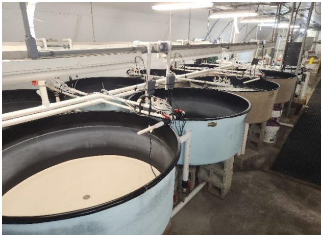
Figure 42. Commercial scale RAS based larviculture tanks for warm water marine fish with pelagic eggs and larvae.
