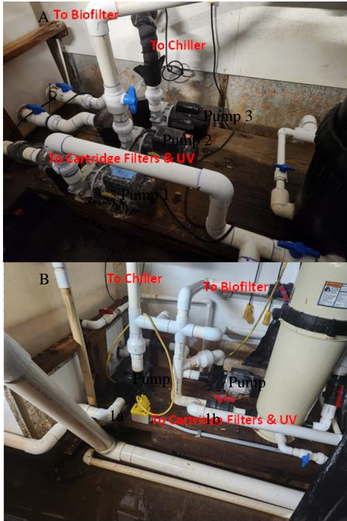
Figure 17. Photos showing two system plumbing designs currently being used at HBOI for Broodstock conditioning systems; A) design as depicted in Figure 16 using three pumps each operating its own loop, B) modified design as described in text using two pumps operating all three filtration loops.
