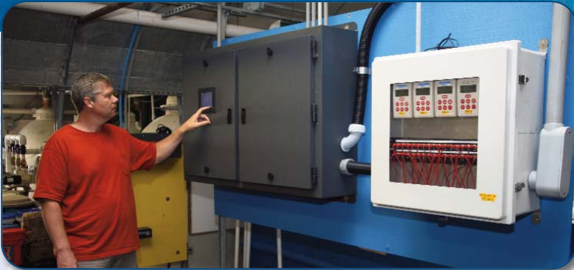
Paul Wills can check the oxygen levels in his research tanks from any computer in the world using the system that he and USDA/ARS aquaculture engineer Tim Pfeiffer designed and built.
