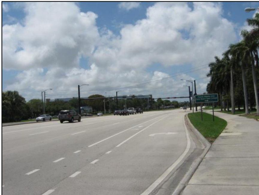
GLADES ROAD – VIEW FACING WEST
