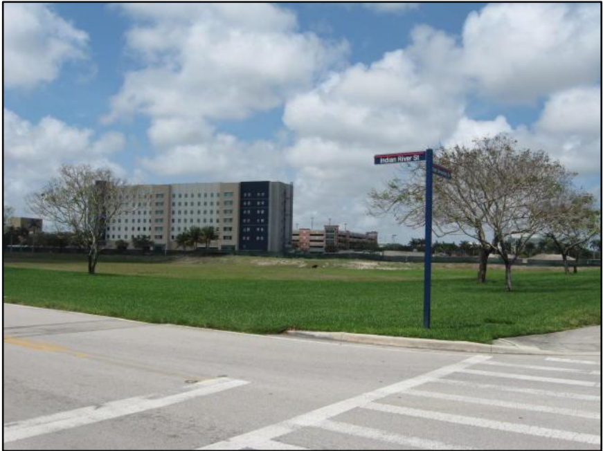
NW QUADRANT – VIEW FACING NORTHWEST
