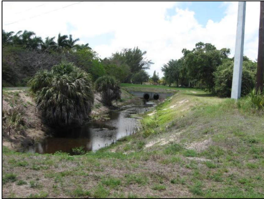
SE QUADRANT – VIEW OF DRAINAGE CULVERT ALONG SOUTH SIDE, FACING SOUTHWEST
