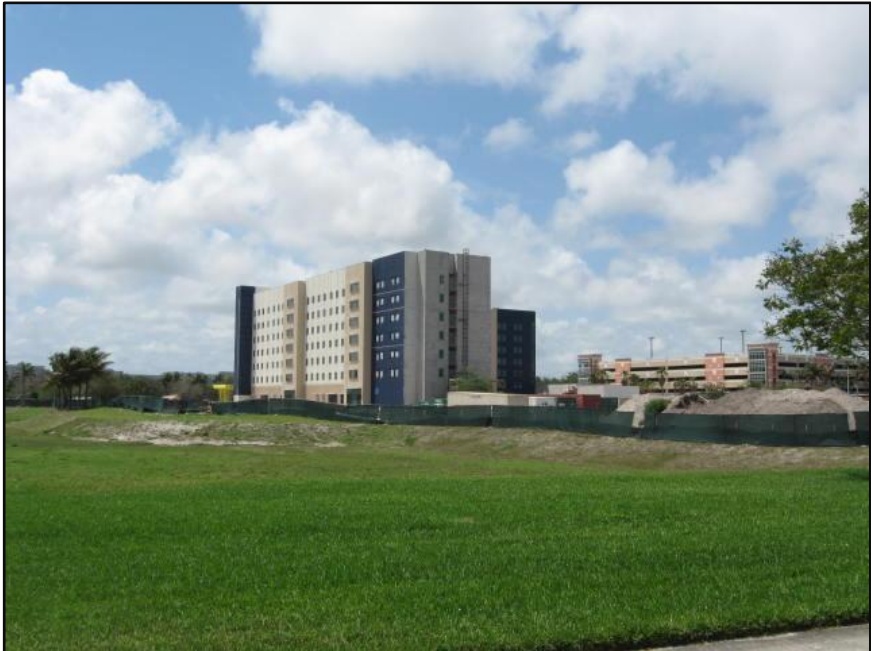
NW QUADRANT – VIEW FACING NORTHWEST ALONG NORTH SIDE
