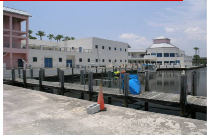
6. View at SE corner looking SW at FAU buildings
