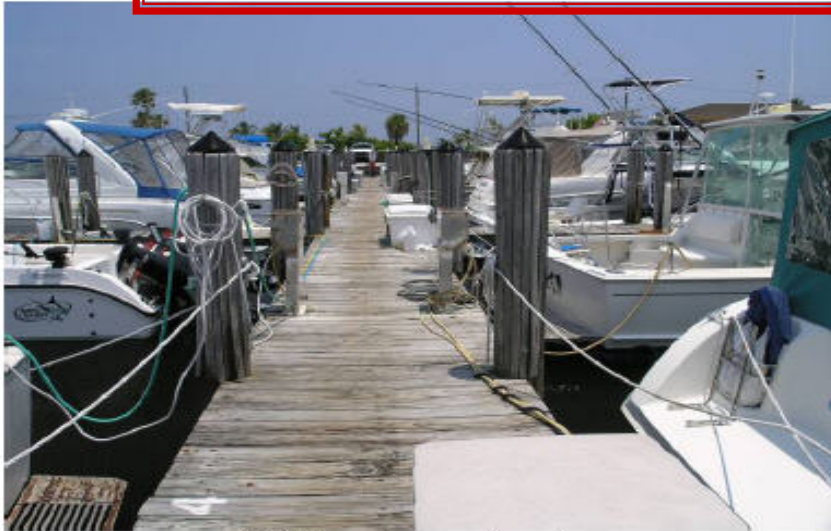
9. View along center pier
