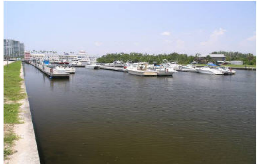
2. View looking south at floating docks
