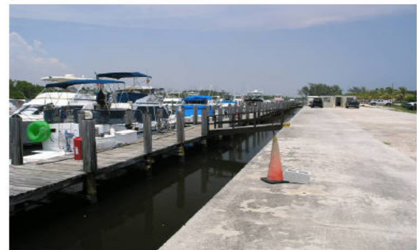
8. View north from SE corner
